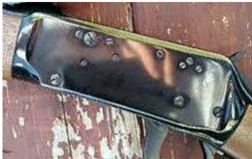
Factory drilled side mount holes on the models 54 and 100. Note there are the standard factory drilled receiver sight holes as well. (Author photo)
